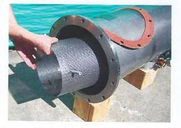
Figure 13: Removal of prestrainer.
